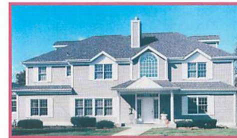
Jarro Building Industries Corp.
